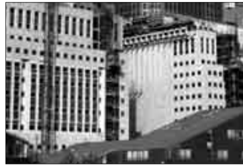
Office Construction in the CBD, Frame and panel
