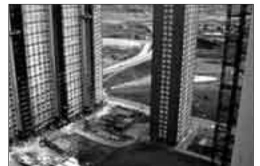
32 storey housing, prefab concrete frame and panel
